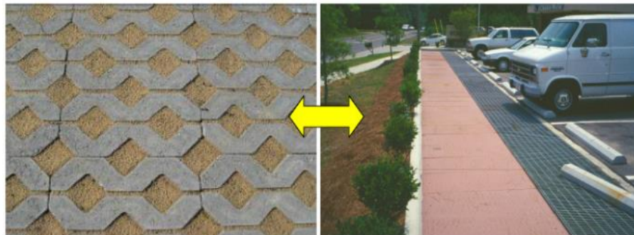
Figure 1.2: Typical Modular permeable pavement design: lattice type (left) and castellated type (right). Source: Whipple (1982)
